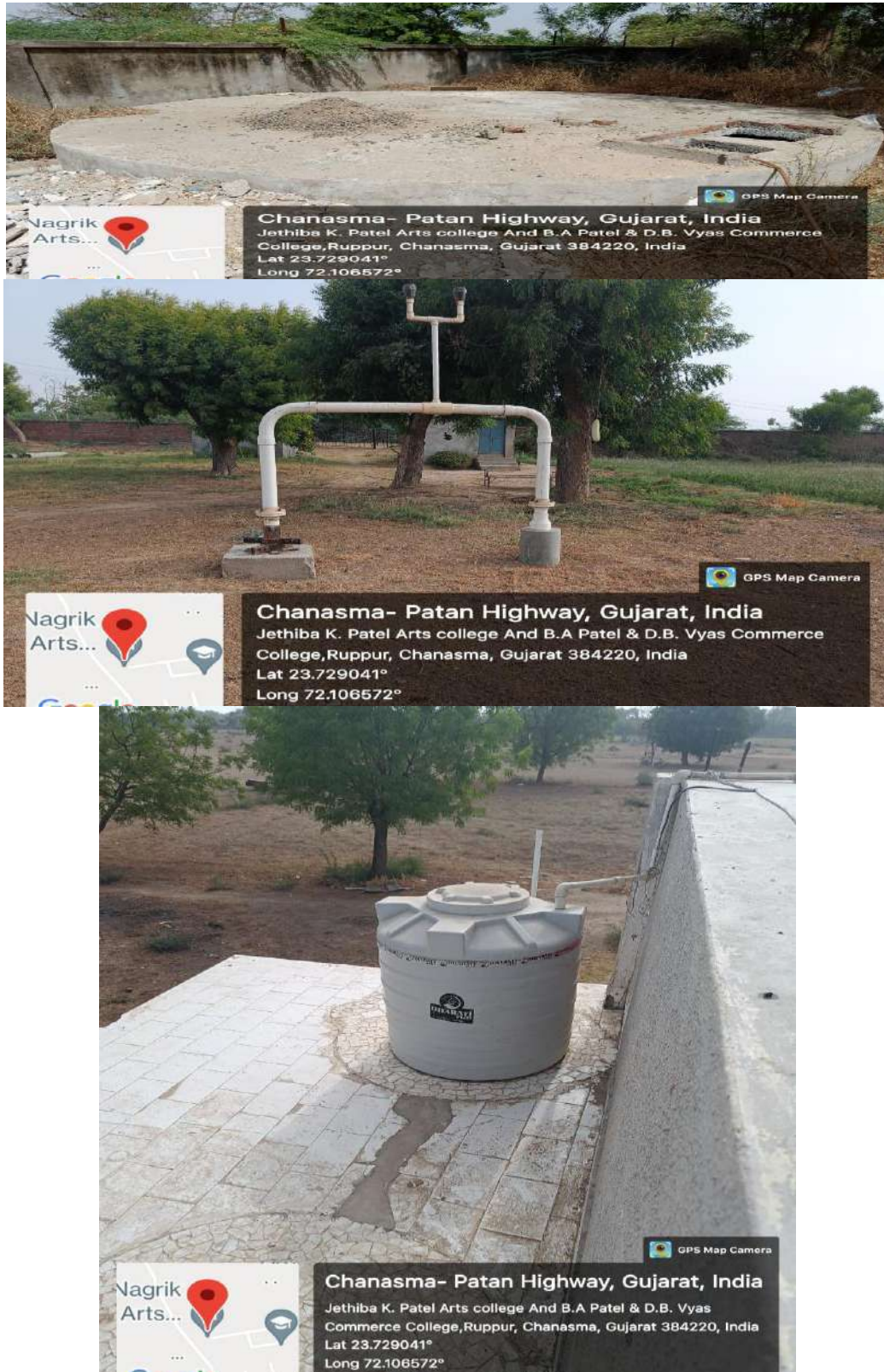
Photo – Storage Water tank
