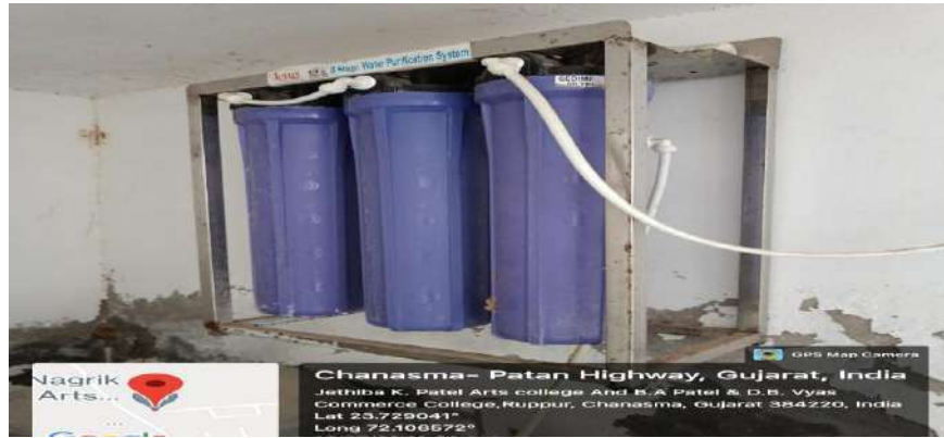
Photo – Ro water purifier and water facility
